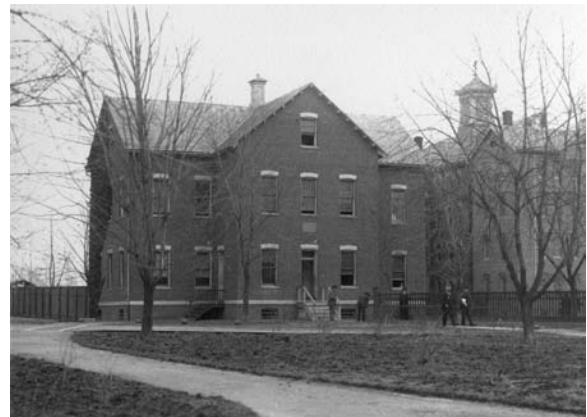
Figure 10. View of Atkins Hall from the west, with Relief beyond at right, circa 1896. Source: 1896 Annual Report and GSA archive, image DC1343SE0P009.
