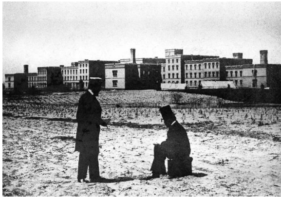
Figure 4. Archival photograph from the southeast of the Center Building group, East Lodge, and West Lodge (no longer extant), circa 1861. Source: GSA archives, image DC0066SE0P035.
