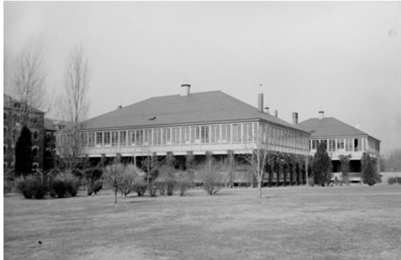
Figure 20. View from the southeast of Allison D with Allison C in the background, 1900. Source: GSA archives, image DC0074SE0P003.
