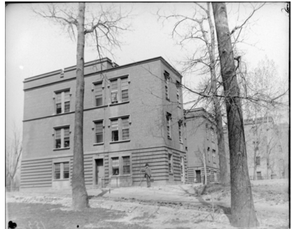
Figure 5. View from the southwest of Garfield, showing lavatory addition, 1898. Source: GSA archives, image DC1441SE0P003.
