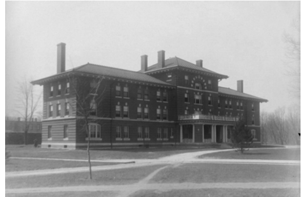
Figure 32. View from the northwest of the E Building, 1905. Source: GSA archive, image DC1465SE0P002.
