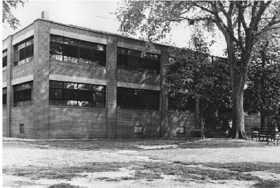
Figure 41. View of Allison D following renovation of the wrap-around porch, 1936. Source: GSA archives, image DC0074SE0P002.
