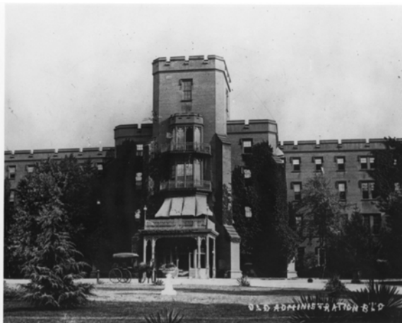
Figure 6. View from the north of the Center Building with porte cochère, balconies, and fourth floor additions to side wings, circa 1889. Source: GSA archives, image DC0066SE0P003.
