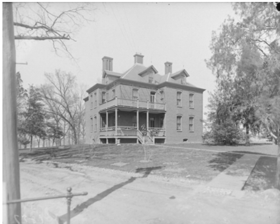
Figure 18. View from southwest of Burroughs Cottage, circa 1897. Source: GSA archive, image DC1447SE0P004.
