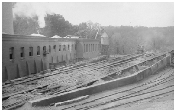
Figure 37. View of north facade of Power House, 1920. Source: GSA Archive, image DC0100SE0P004.
