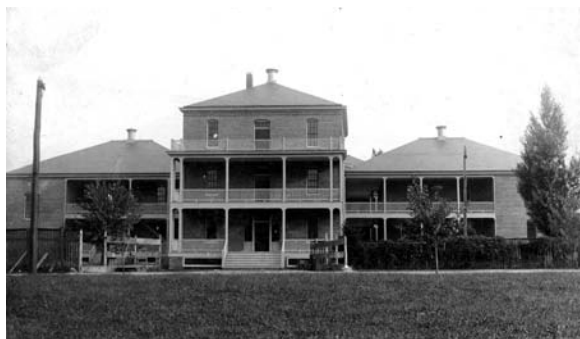
Figure 19. View of the Allison group from the north, nearing completion, September 20, 1898. Source: GSA archive, image DC1450SE0P002.
