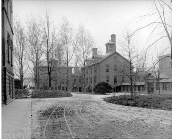
Figure 22. View of the original Bakery building (right side of image) with covered breezeway connecting to the West Wing (Building 3), 1898. Note ventilation stack on roof of 1878 portion of the Bakery. Source: GSA archives, image DC1458SE0P004.
