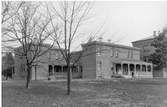
Figure 16. View from the northwest of Linden (left) and Holly (right), circa 1900. The East Lodge /Detached Nurses Home is visible in the background. Source: GSA archives, image DC0148SE0P003.
