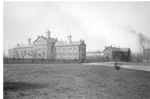
Figure 9. View of Atkins Hall (right), Relief (left), and Detached Dining Hall (background) shortly after their construction, circa 1895. Source: Image 418-H-31; Records of St. Elizabeths Hospital, Record Group 418; National Archives at College Park, College Park, Maryland.
