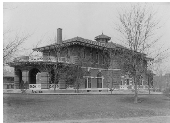
Figure 35. View of the L Building from the southeast, circa 1905. Source: GSA archives, image DC0107SE0P020.
