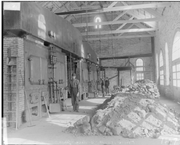
Figure 27. Interior view of the Boiler House/Ice Plant, 1897. Source: GSA archives, image DC0100SE0P002.
