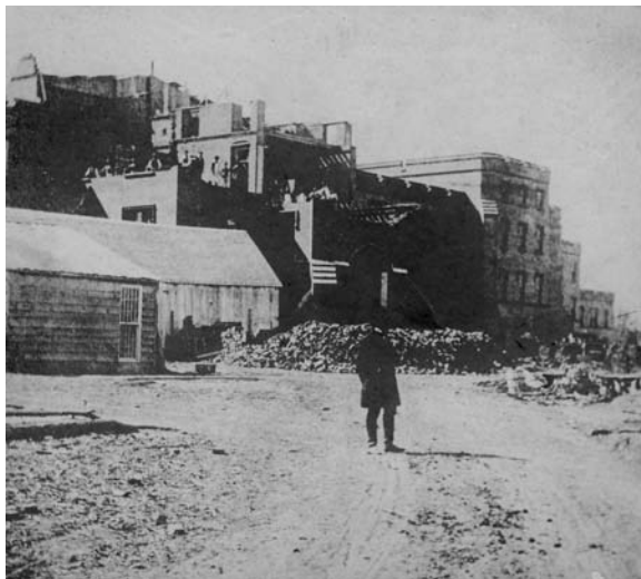
Figure 3. The Center Building under construction, circa 1857–1858. Source: GSA archives, image DC0066SE0P036.
