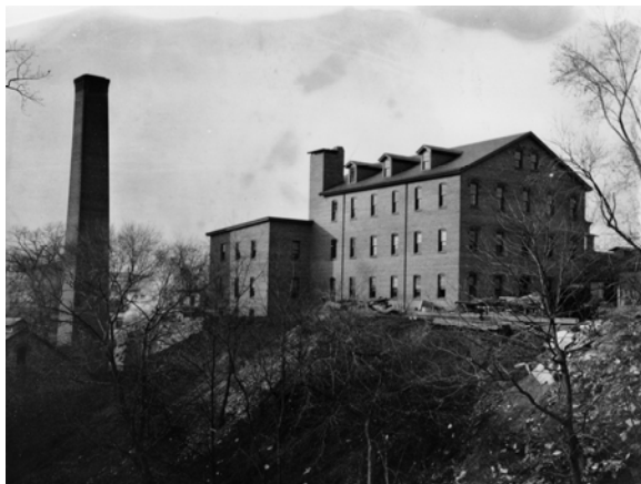
Figure 21. View from the southeast of the General Laundry addition as it appeared shortly after completion in 1899. Source: GSA archive, image DC1472SE0P205.
