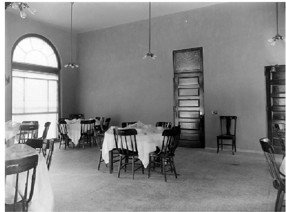
Figure 34. View of the communal dining hall of the K Building, 1905. Source: GSA archives, DC0110SE0P002.
